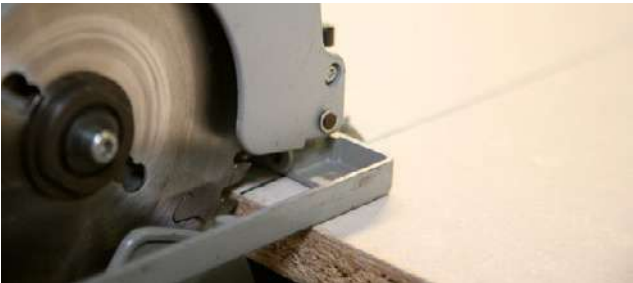
Picture No. 3: Cutting handheld circular saw.
