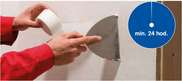
Picture No. 8: Covering of the edges.
