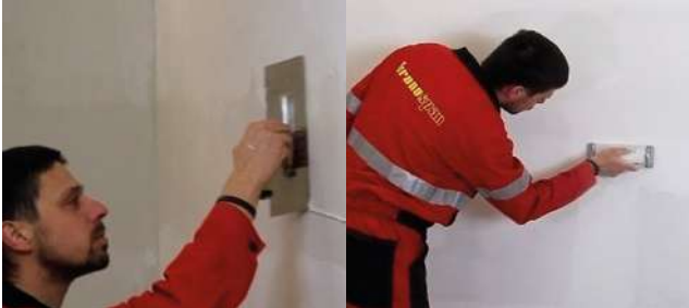
Picture No. 9: Covering of the edges.
