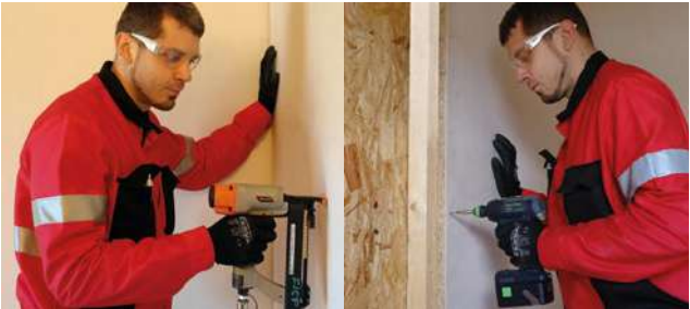
Picture No. 6: Nailing, stapling.
